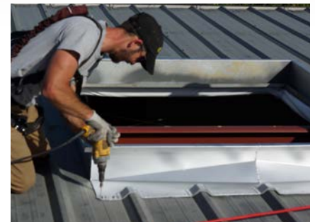
3. Install roof curb.
